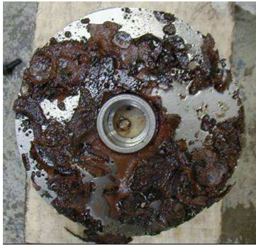
Figure 5.9: Varnish and plastic from windings deposited at the bottom of the compressor
