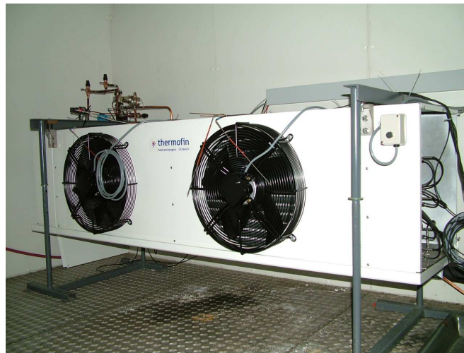
Figure 4.17: View of rib evaporator cooling cell
